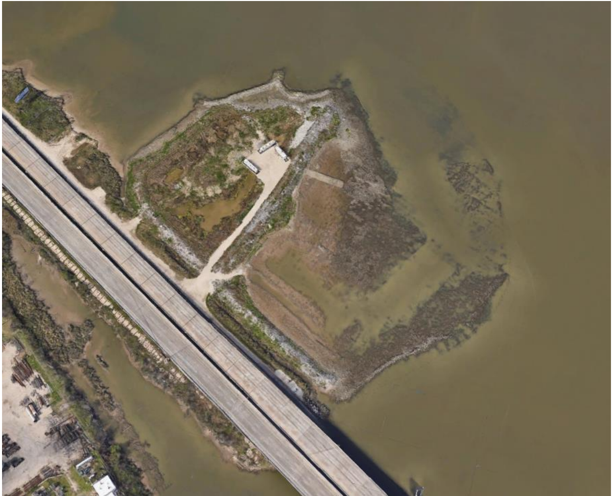
The Northern Pit is now partially submerged in the middle of the San Jacinto River, Channelview, TX (Google Earth).
