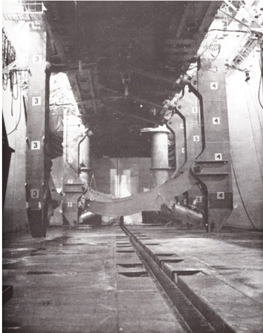
“Clementine” inside the HMB-1, showing the flap doors in the floor that would open to allow the claw to be lowered to the seafloor.
