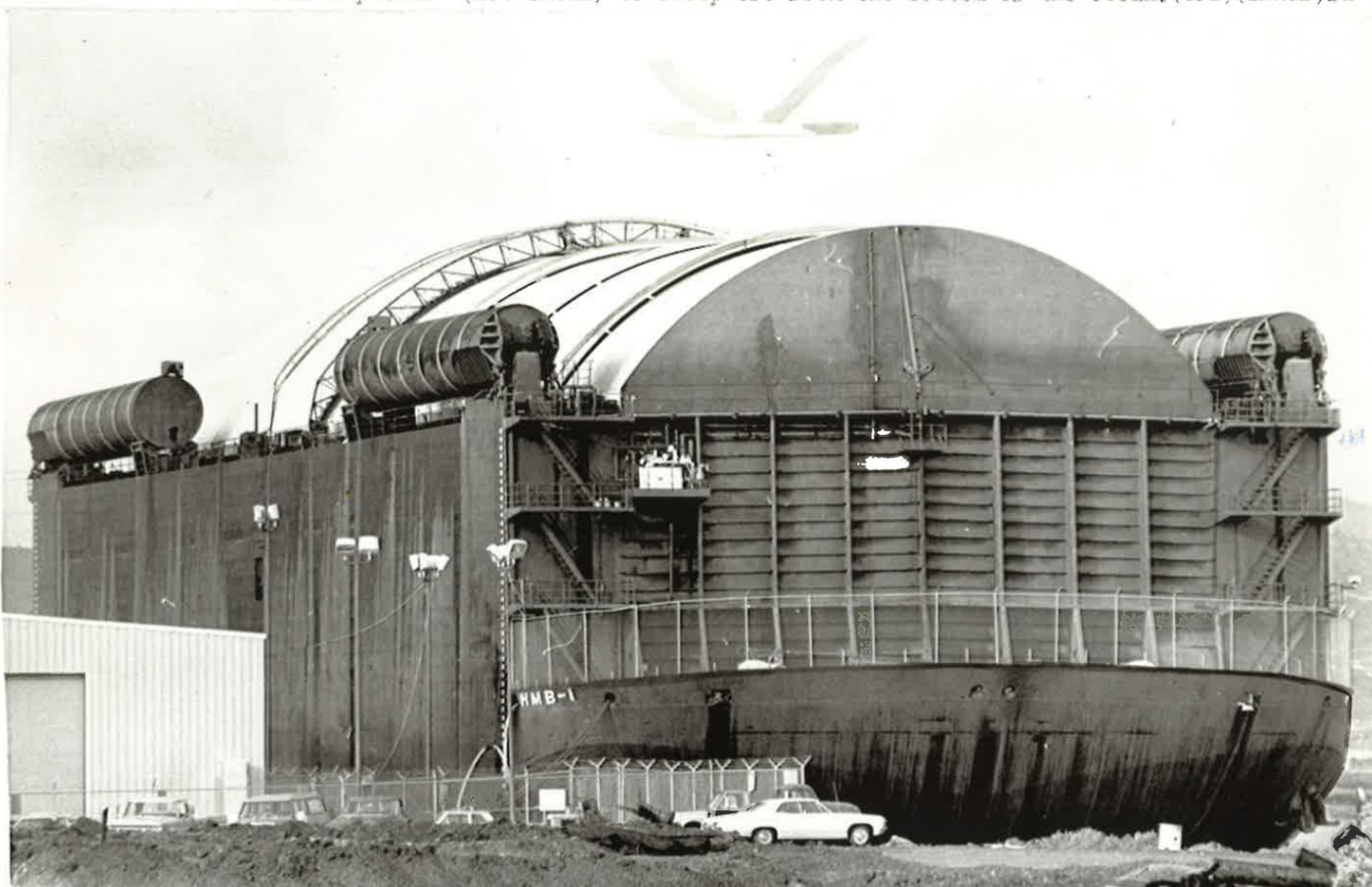
The Hughes Mining Barge (HMB-1) prior to Project Azorian, with the caption giving the cover story. January 6, 1974.
